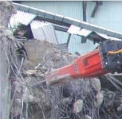
Heavy duty demolition
