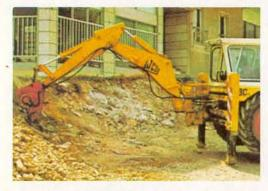
Rapid-Ram is an ideal hammer for cleanup operations where its mobility and performance make the job go faster and more economically compared to workers using hand-held pavement breakers and their companion air compressor.
