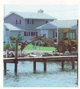
The versatile Rapid-Ram handles dozens of demolition jobs more economically than workers with hand-held air breakers and the necessary compressor.
